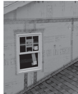
■ Figure 4. FPIS WRB System installation using joint tapes and adhered flashings; refer to manufacturer installation instructions for specific details.
