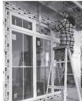
■ Figure 4. FPIS WRB System installation using joint tapes and adhered flashings; refer to manufacturer installation instructions for specific details.
