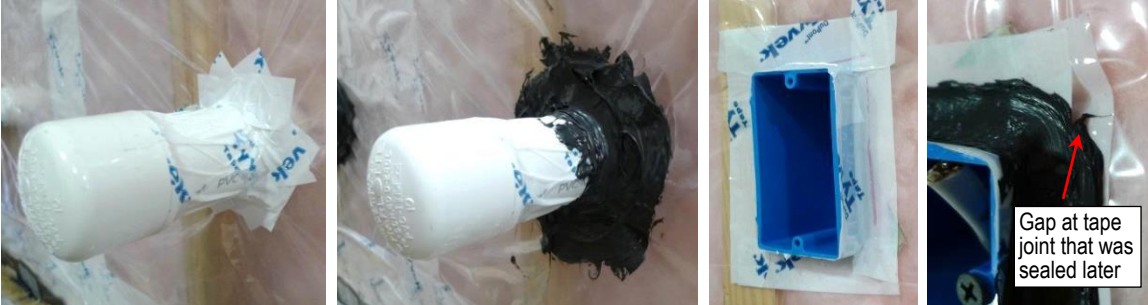
Figure 16. Penetrations through membrane sealed with tape and sealant.
