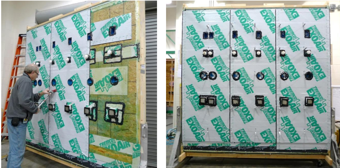
Figure 28. Test wall with asphalt-based, self-adhered membrane as the air barrier material.
