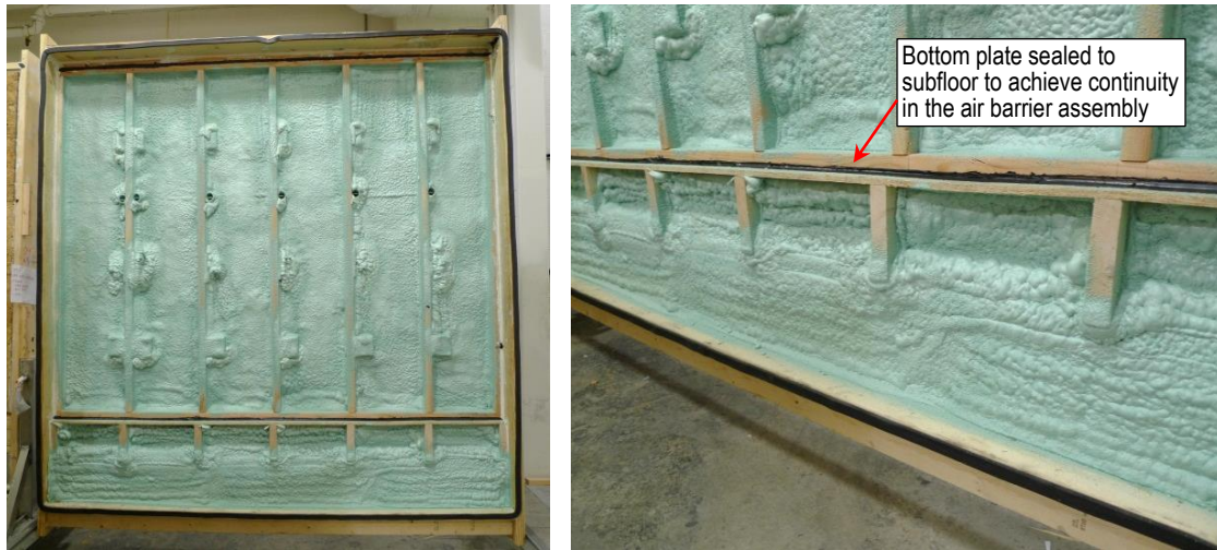
Figure 32. Test wall with 1” closed-cell foam as the air barrier material.
